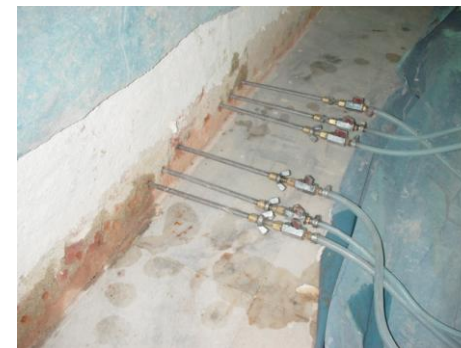
Figure 3. Treatment of a Course of Damp-proofing Through Chemical Injection
