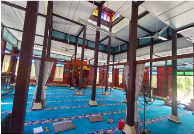
Figure 1. Timber columns at main prayer hall in Masjid An Nur
