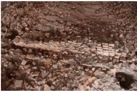
(a) Wall remains in site SB1A
